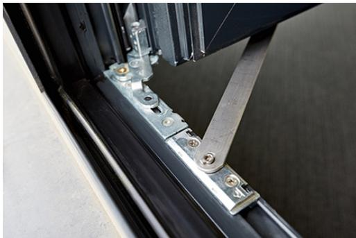
The window fabricator equipped the opening elements in THE GRID with fully concealed, horizontal 'Roto AL Designo' range hardware and also a lockable opening restrictor. Puristic design and efficient utilisation are guaranteed by this combination.
