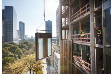
The facade manufacturer FKN produced facade elements and 4293 Turn-Only window sashes, equipped with the “Roto AL Designo” premium hardware, for the Marienturm in the banking metropolis of Frankfurt.
