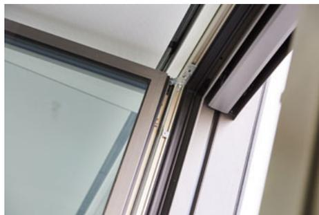
For the Turn-Only windows on the Frankfurt Marienturm, the Roto Object Business developed four hardware configurations consisting of components from the “Roto AL Designo” fully concealed Tilt&Turn hardware product range depending on the weight of the sashes..
