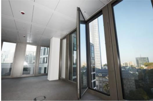
The facade specialist FKN used four versions of the “Roto AL Designo” hardware for the Frankfurt Marienturm’s Turn-Only balcony doors with a sash weight of up to 180 kg.
