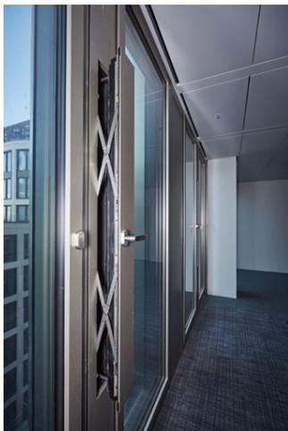
The inward-opening ventilation flaps on the Frankfurt Marienturm feature parallel projecting scissor stays from the “Roto PS Aintree” product range and Roto special corner drives. When open, the ventilation flaps in the facade manufactured by FKN ensure an extremely high air exchange rate.
