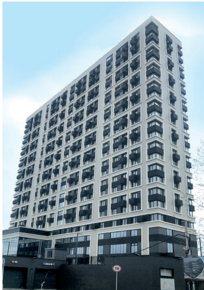
In the "Love and Pigeons" residential building in Moscow, 580 Tilt&Turn windows by the window specialist Schtandart ensure light and ventilation for the interior.
